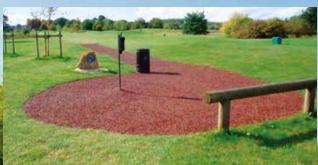
TigerTrak is mixed up and wet-laid on site, forming an in situ surface that is incredibly strong. As the rubber is bound with the polyurethane, the shreds do not move out of place, providing a strong and durable surface. The overall effect is to create a highly decorative surface that will do its job for many years. When laid TigerTrak is slightly soft underfoot, making it a comfortable surface for pedestrians and strong enough to accommodate buggy traffic.
