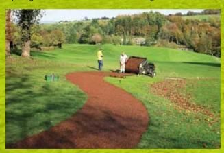
Ease of installation means TigerTrak can be laid to form new paths or overlaid on to existing hard surfaces, such as hoggin, MOT1 or green shale. We recommend that new installations are laid on to a suitable sub base of compacted free draining aggregate. The depth of this will vary according to ground conditions.
